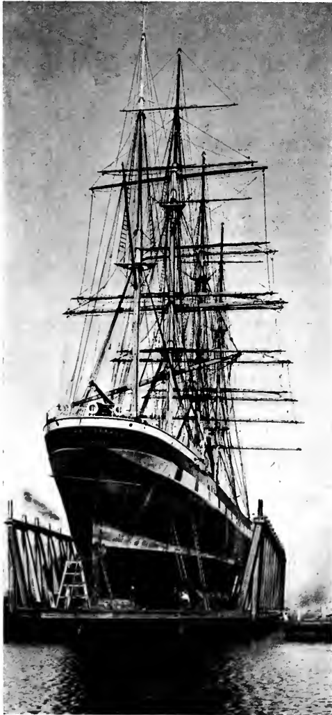
The "Crown of Germany" on a 3,000-ton Crandall dock at Victoria, B. C. This dock is of composite construction.
